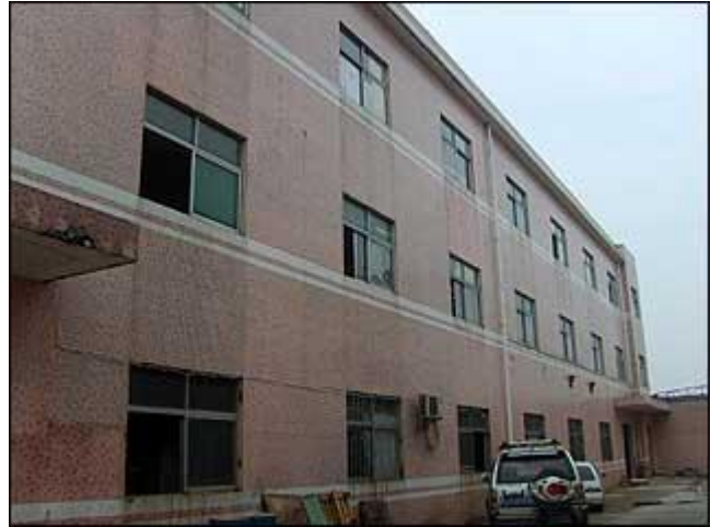
Factory exterior view
